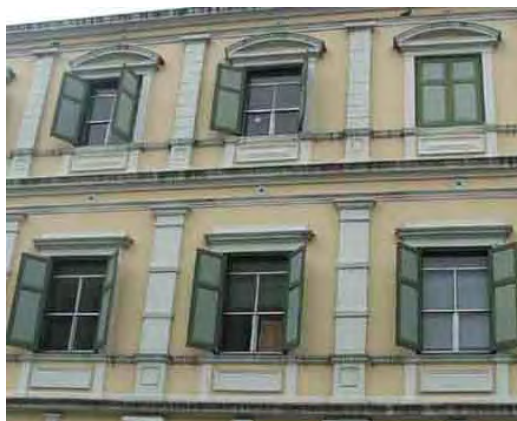
Figure 18. Aluminum window frames are installed / Building A.
