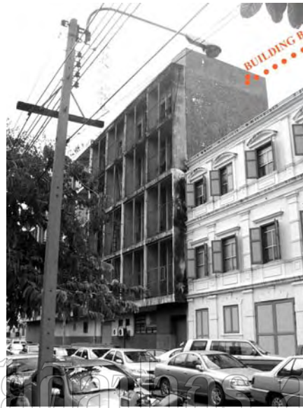
Figure 9 and 10. Building C / Ministry of Defence.
