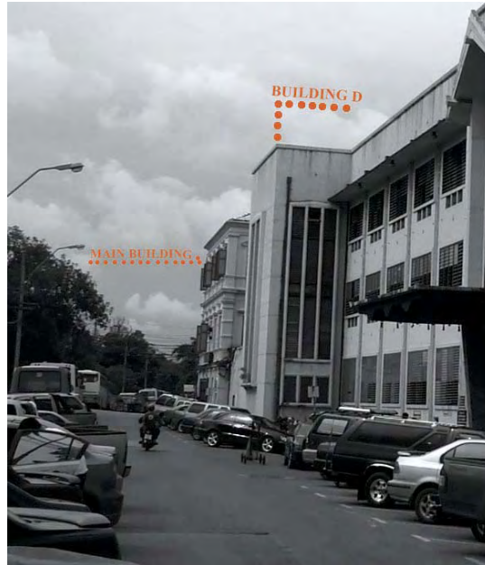
Figure 12. Building D / Ministry of Defence. (photo: Mr. Korn Prabhasabhakdi, 2005)
