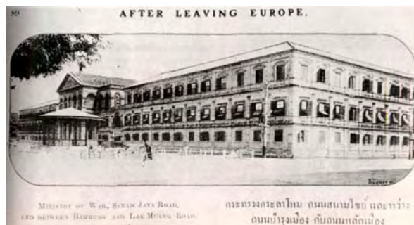
Figure 7. Building A / Ministry of Defence.
